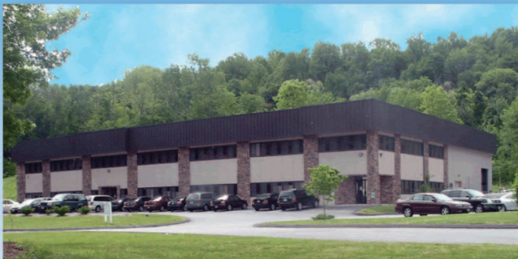
EE Controls Home Office Brewster, NY
